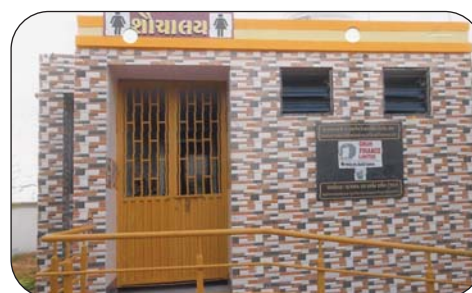
GRUH provided funding for construction of Sanitation Units at Dist. Surendranagar, Gujarat.
